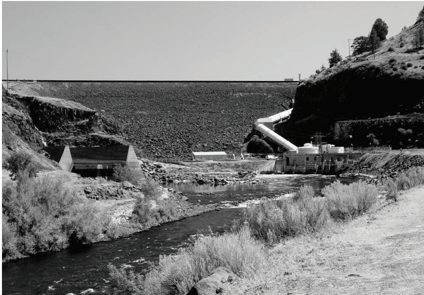
FIGURE 1-2 Iron Gate Dam on the Klamath River is the dividing point between the upper and lower Klamath River basins. The penstock for the power generators is on the right, and the spillway is on the left in this view looking upstream.
