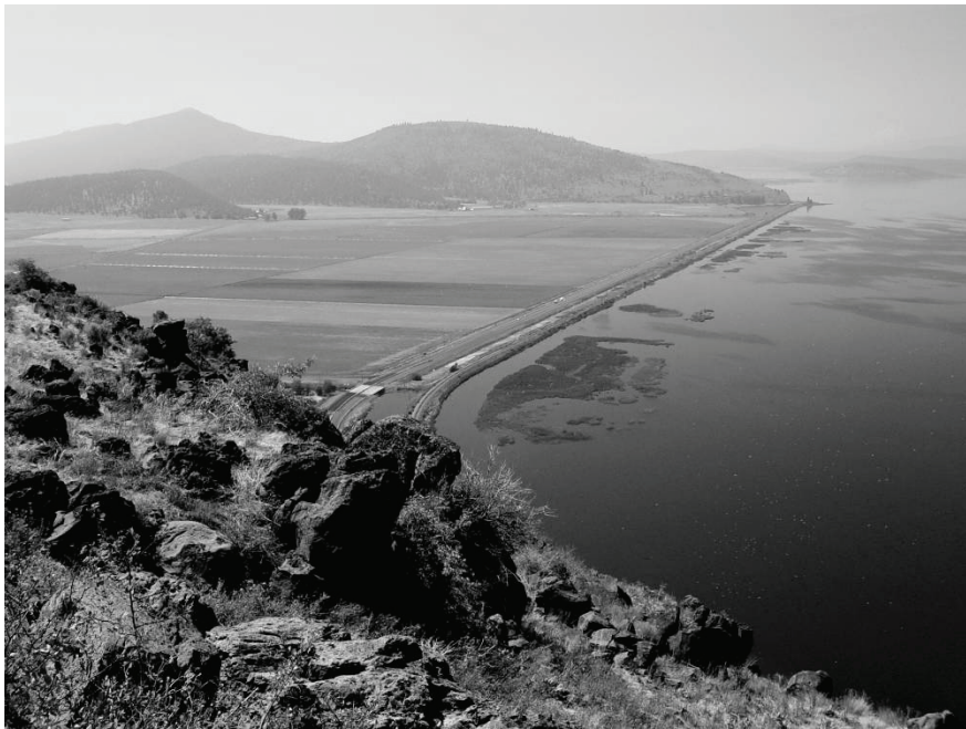
FIGURE 4-6 The NFS adjusted flows from the upper Klamath River basin to account for the conversion of marsh areas to agriculture, such as shown here on the southeast side of Upper Klamath Lake. Levees separated the area now under cultivation (on the left) from the lake and its marsh area (on the right).
