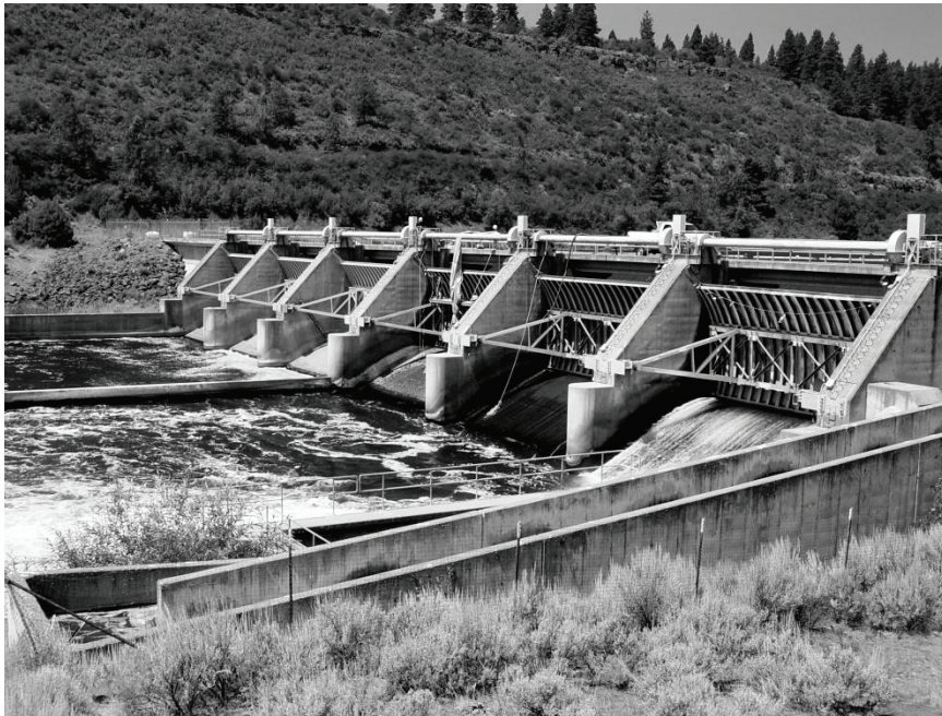
FIGURE 4-1 Keno Dam rests atop a bedrock sill across the Klamath River near Keno, Oregon. The fish ladder for the dam is on the left abutment of the dam in the foreground of this view.
