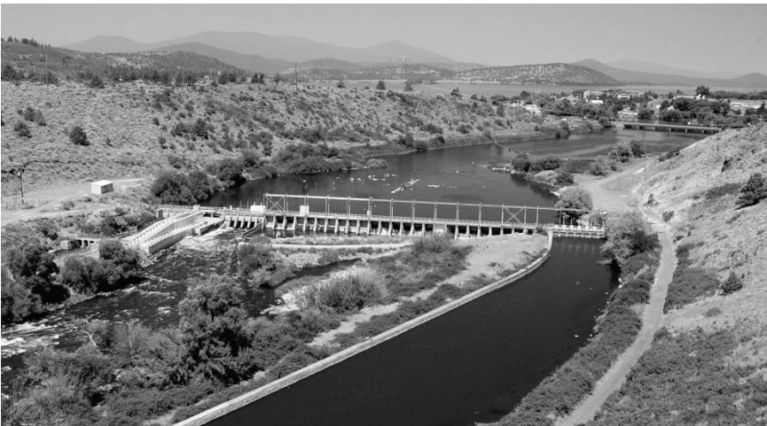
FIGURE 2-2d The Link River Dam, shown in this 2006 view from the same location as the views in Figures 2-2 a, b, and c, now includes a fish ladder, recently installed near the right abutment (left side of the dam in this image).
