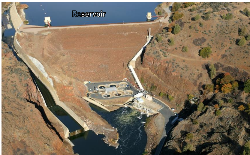
Figure 4.2-16: Photo of Iron Gate Dam and reservoir with specific components labeled. With full facilities removal, all visible components would be removed. With partial facilities removal, certain components (e.g., penstock) would be retained.
