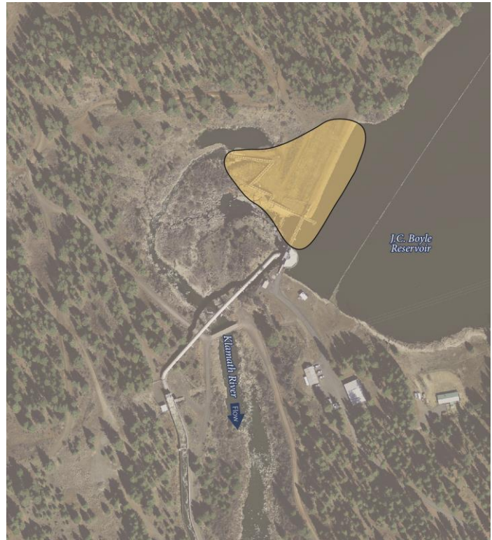
Figure 4.2-5: Partial removal of the J.C. Boyle Facility would provide a free flowing river and allow full volitional fish passage. However, certain structures would be retained.
