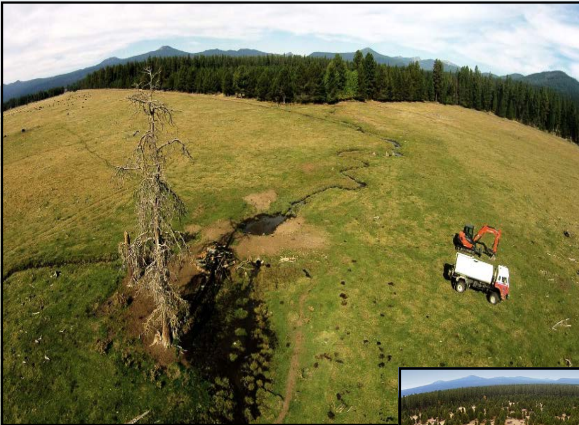
Beginning the reconnection process along Sun Creek's historic channel in a forested portion of the watershed
