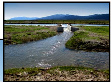
Constructed fish bypass channel
