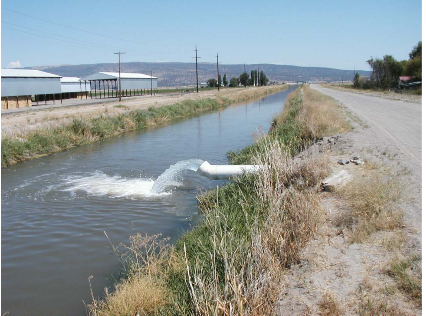
Figure 3-11. Water is moved to areas of need by way of diversion canals such as this one in the Tule Lake subbasin. (Photograph by Charles Palmer, USGS.)
