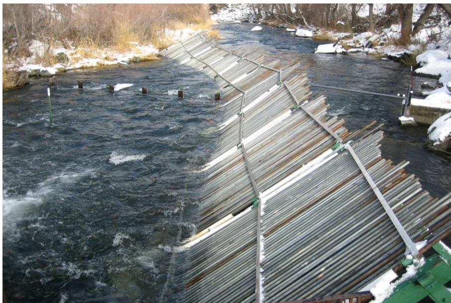
Figure 2. Alaska-style panels of the Shasta River Fish Counting Facility (SRFCF)
