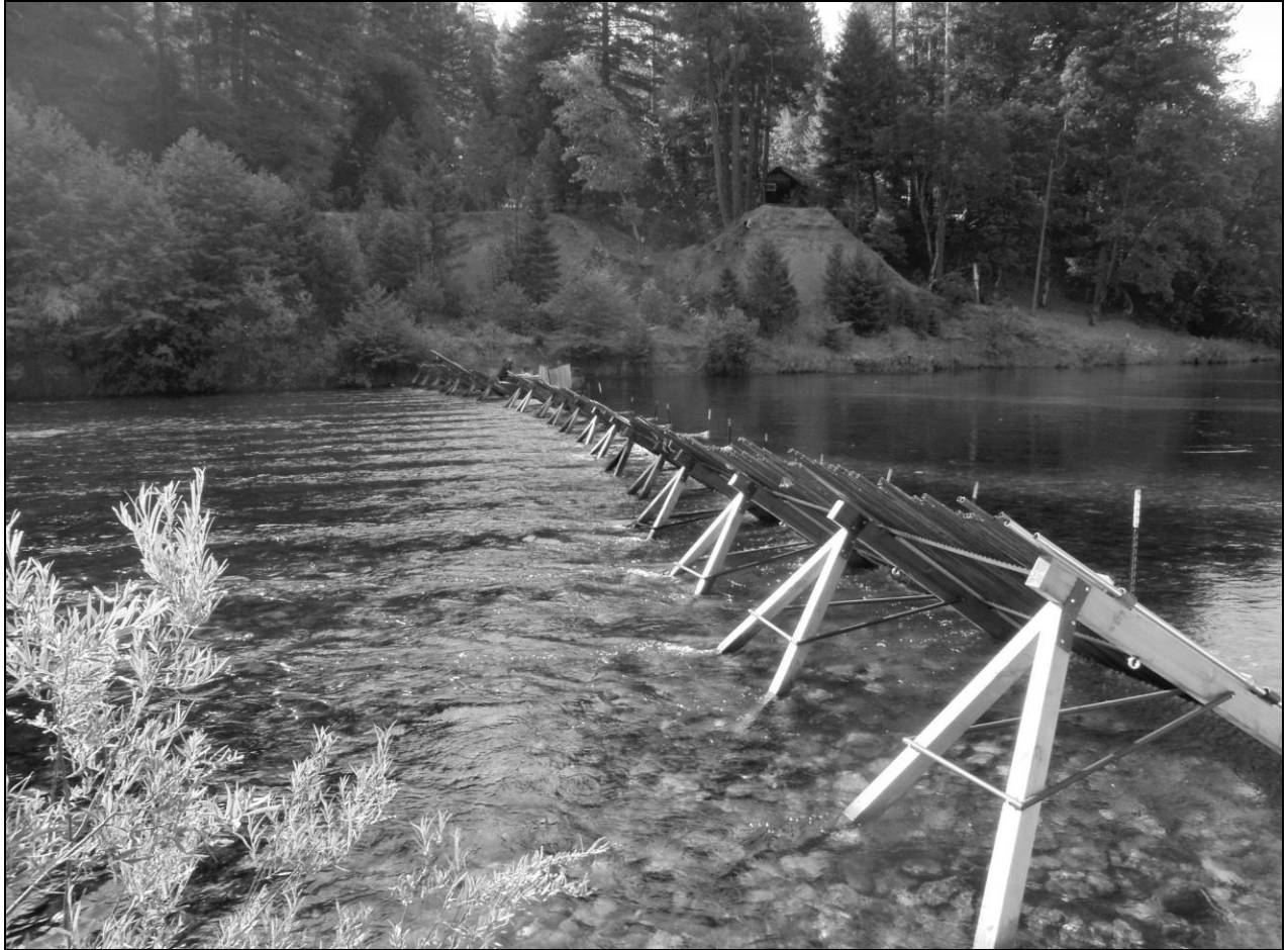
Figure 4. 2013 Junction City weir configuration (looking slightly upstream). Note the single trap box (on far side).
