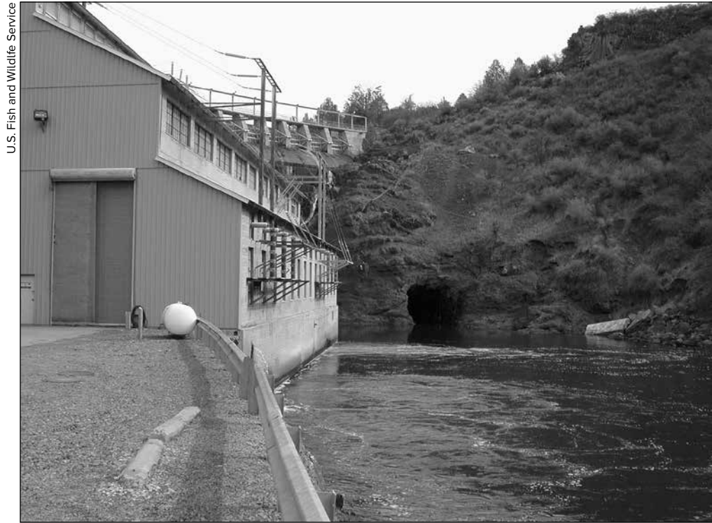
THE TUNNEL used to divert the Klamath River during the construction of Copco 1 Dam is still apparent. This photo was taken in 2003.
