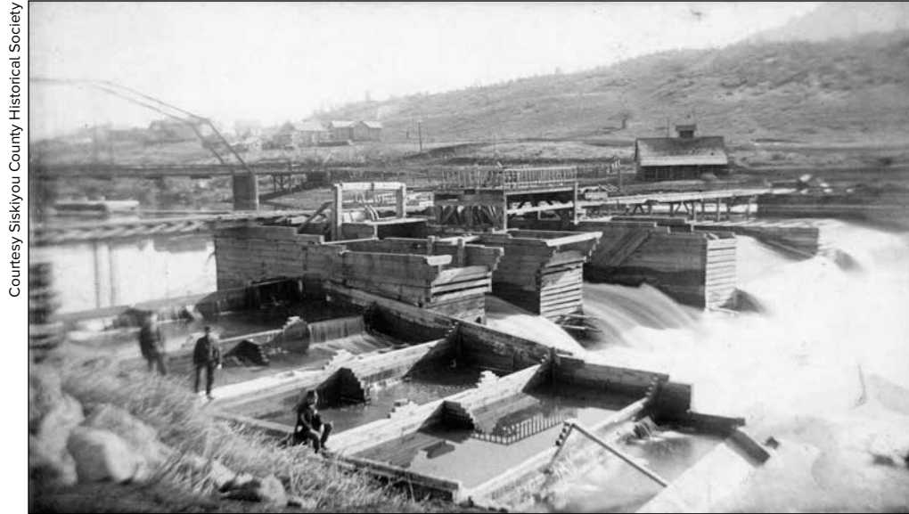
THE REBUILT KLAMATHON MILL log-crib dam and fish ladder is pictured here in 1892. The original 1889 dam did not provide a path for fish passage, and many salmon died downstream or were captured and illegally sold.
