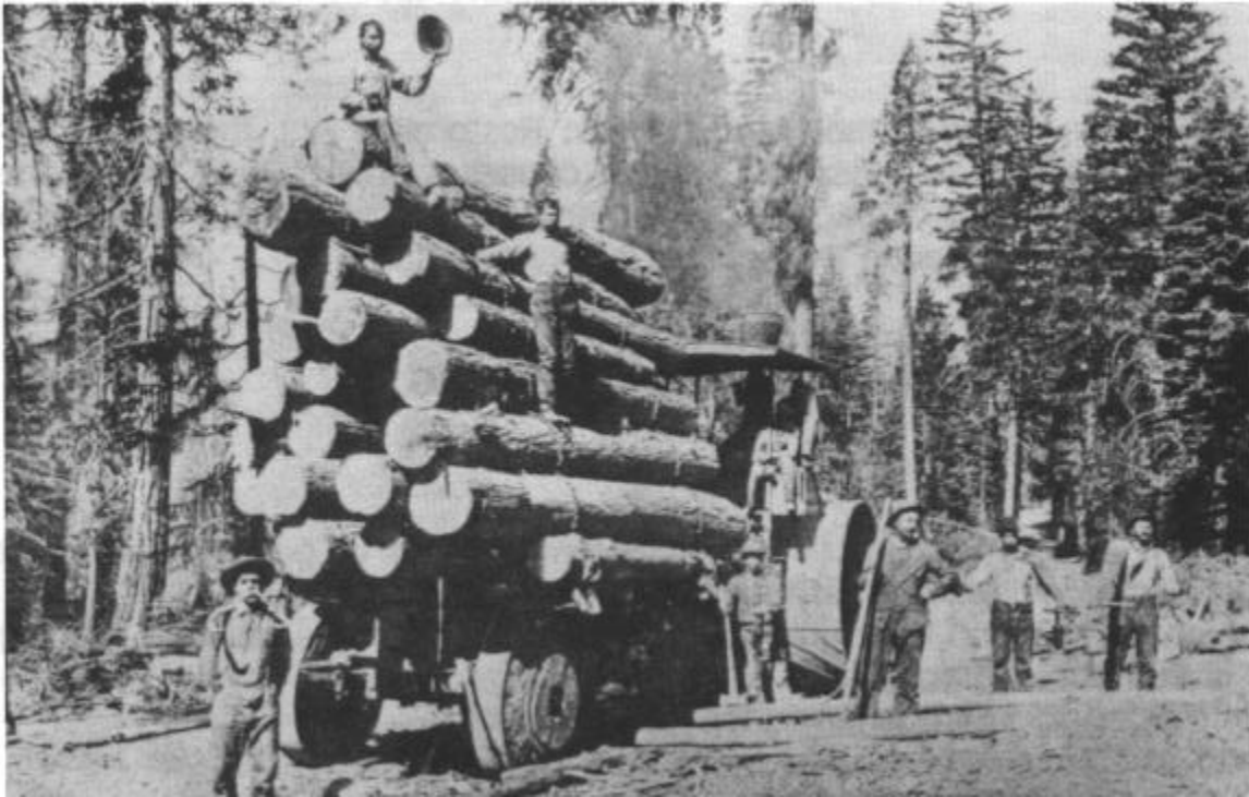
A wooden-wheeled logging cart pulled by a steam donkey.
