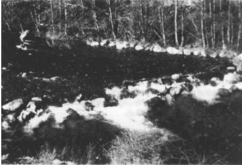
Figure 3-5 -- These boulder weirs on the South Fork of the Salmon River have attracted spawning chinook salmon and steelhead, and also provide rearing habitat.
