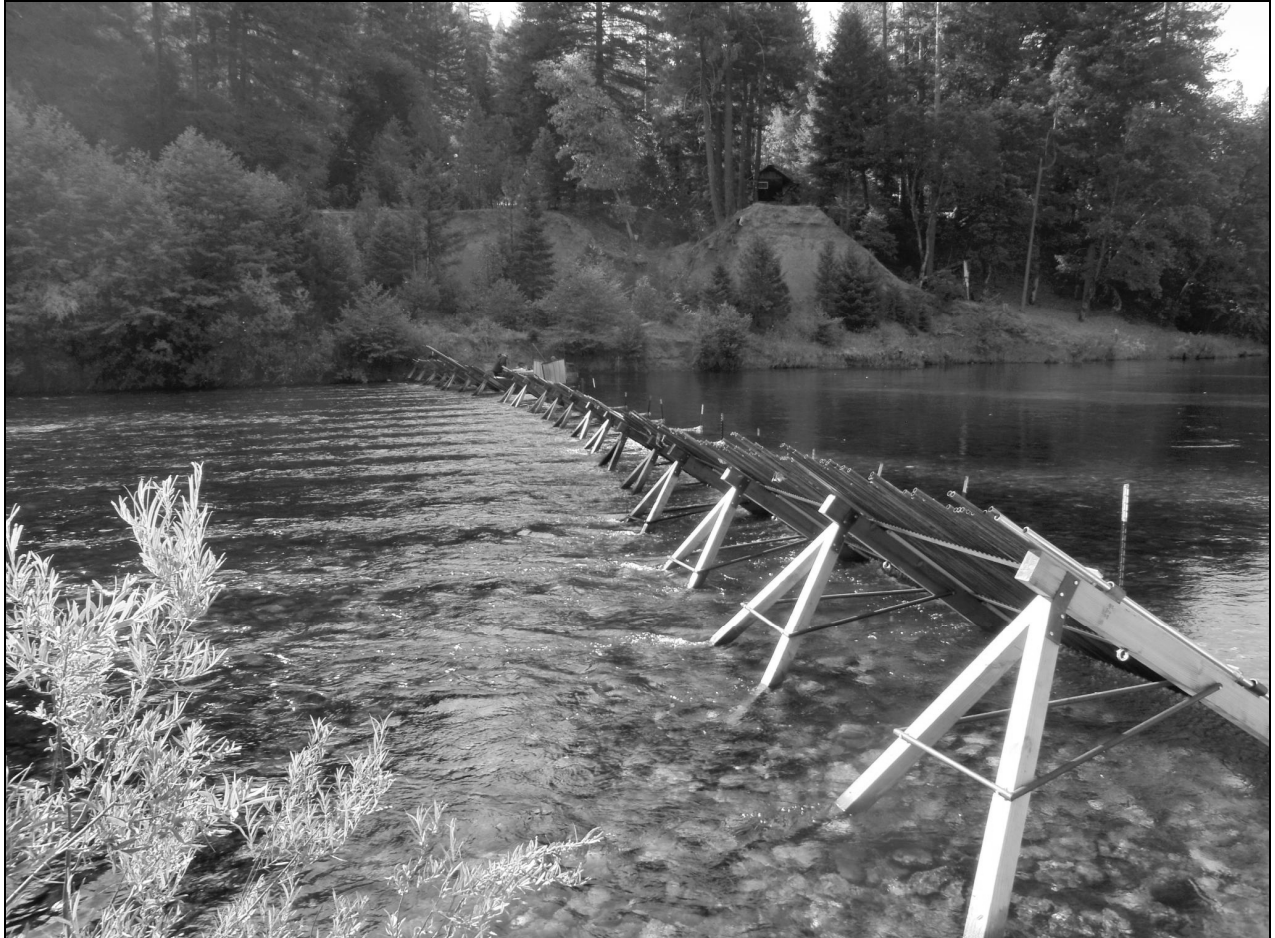
Figure 4. 2014 Junction City weir configuration (looking slightly upstream). Note the single trap box (on far side).
