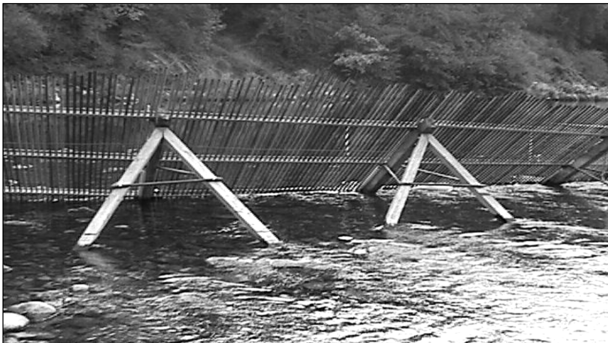
Figure 2. Photograph of Alaskan-style weir, tripods, support channels and conduit (looking upstream).
