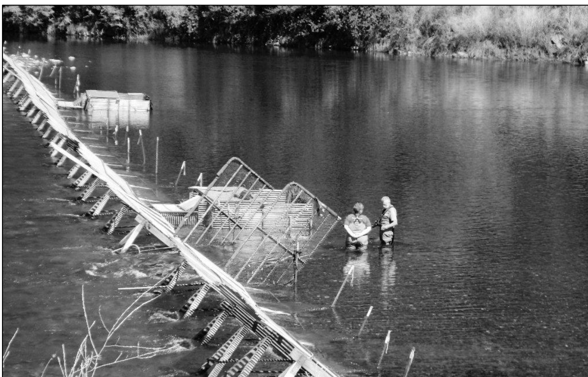
Figure 3. Set up of Willow Creek weir, 2014. Two trap boxes and a boat gate (in opened position).
