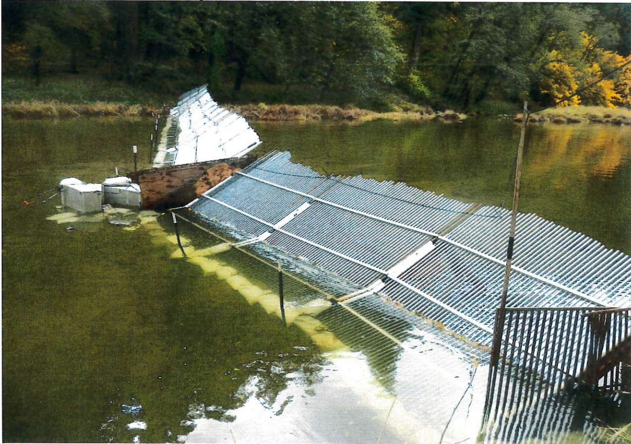
Figure 2. Scott River Fish Counting Facility located in Siskiyou County, California 2015.
