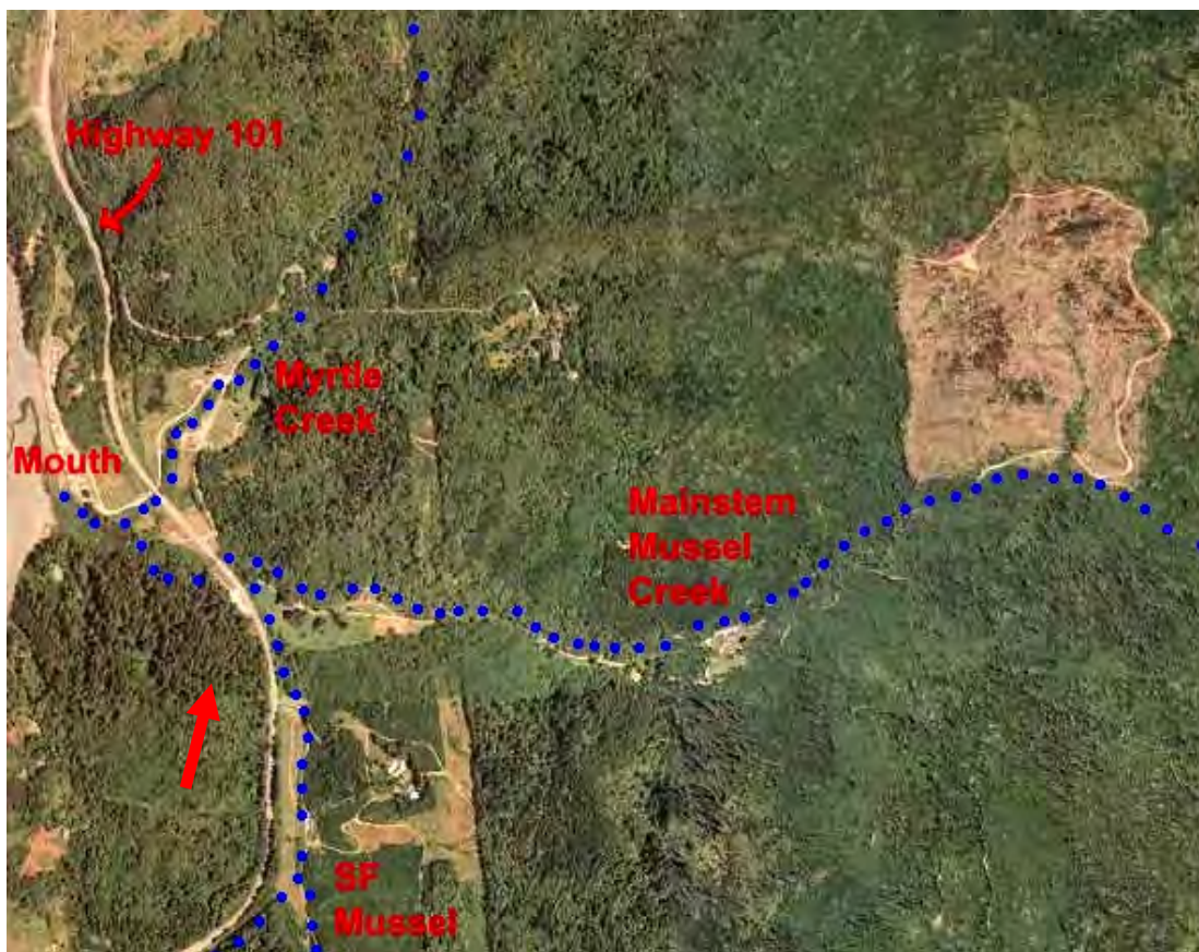
Figure 9-3. The lower reaches of Mussel, South Fork Mussel and Myrtle creeks in June 2005. Note the power line corridor in upper Myrtle riparian, Highway 101 confining South Fork, and a clearcut upper mainstem Mussel Creek. Arrow at lower-left points to patch of large trees, possibly old growth.
