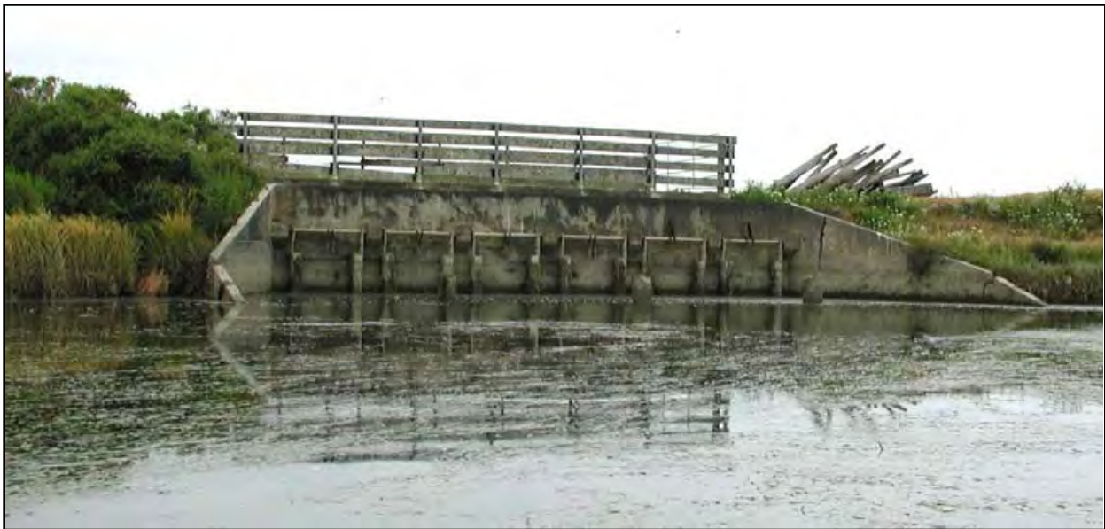
Figure 26-4. Photo of a tidegate on Cutoff Slough in the Lower Eel River estuary.
