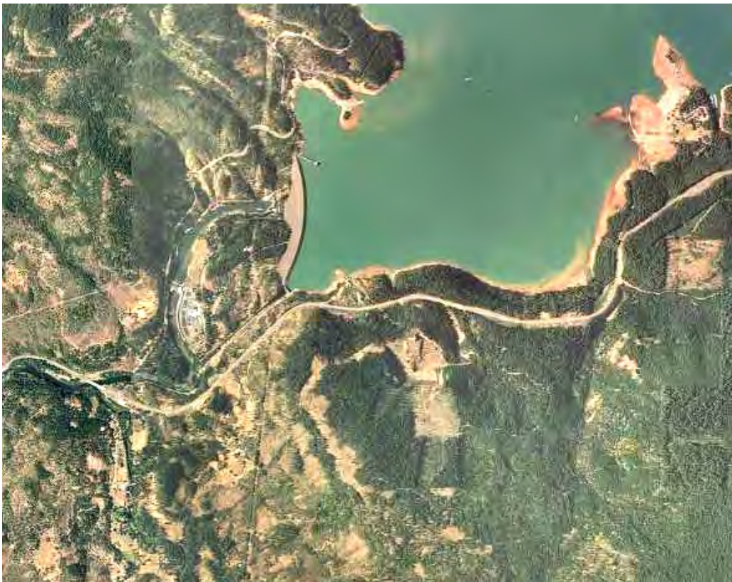
Figure 32-2. William L. Jess Dam. The dam blocks anadromous fish access upstream, but provides a perennially cold mainstem Rogue River flows below the dam (at center left). Aerial photo from June 2005.
