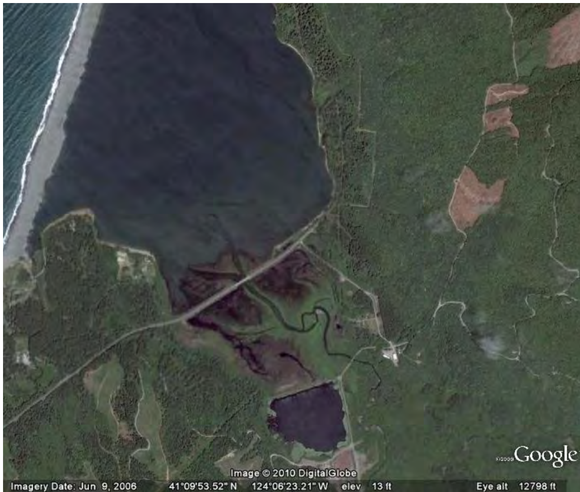
Figure 20-2. Photo shows Gray Creek mill pond and channelization of Maple Creek. Note the reduction of tidal exchange as a result of Highway 101.
