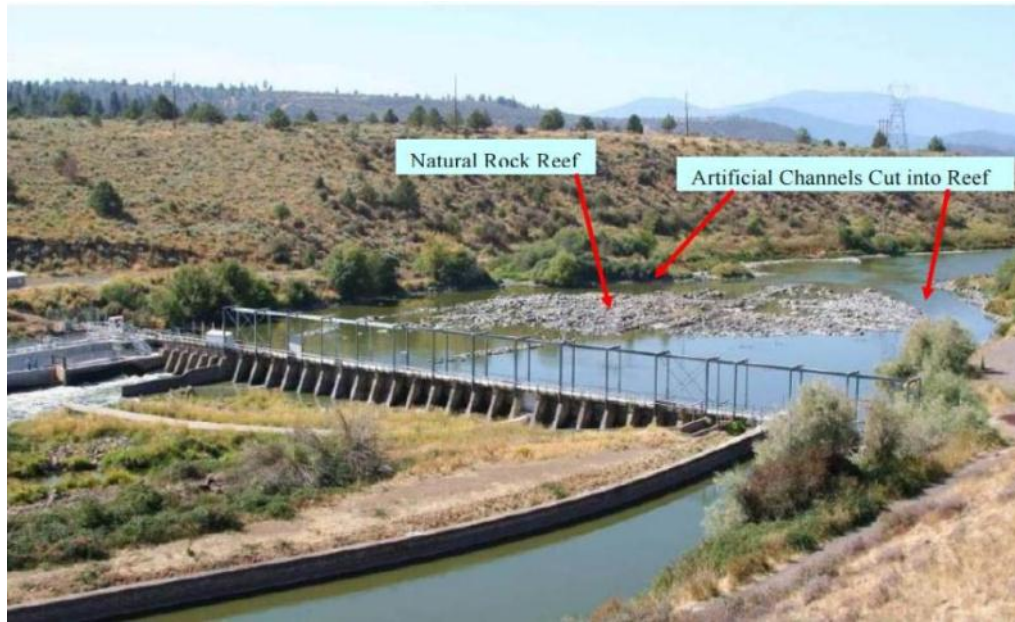
Figure 10. Photo of Link River Dam looking upstream towards Upper Klamath Lake showing the natural rock reef and two artificial channels that were cut through the reef to allow Upper Klamath Lake to be lowered below the historic reef elevation. Source: USFWS 2008.
