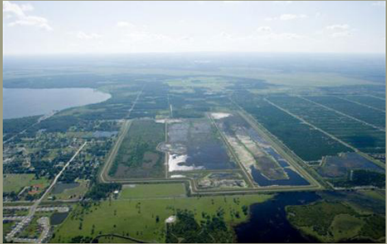
Fig. 2.20 Lake Trafford dredged sediment settling area. Photo: Atkins.
