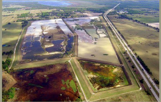
Fig. 2.21 Lake Panosofkee dredged sediment settling area. Photo: Atkins.
