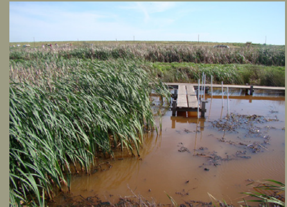
Fig. 3.13 (Below) LICD wetland system for enhanced removal of dissolved organic carbon and mercury in the Sacramento-San Joaquin River Delta, California. Photo: Philip Bachand.
