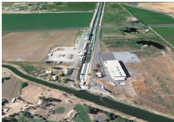
Fig. 2.12 Aerial view of a land-based screen filtration operation. Photo: Google Earth.
