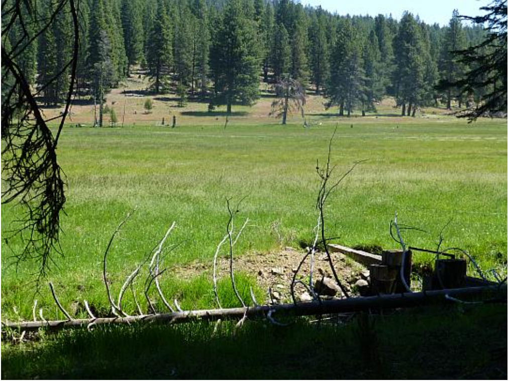
Figure 5. Bull Meadow diversion structure
