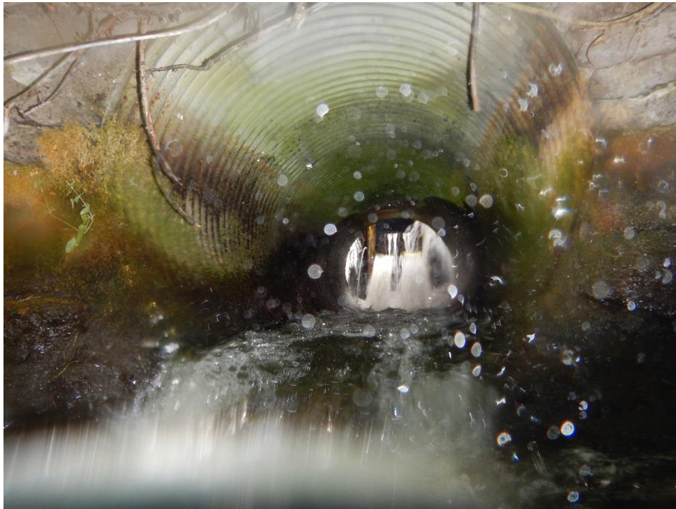
Photo 38. Looking upstream into the culvert from Big Springs Lake, 8-21-14.
