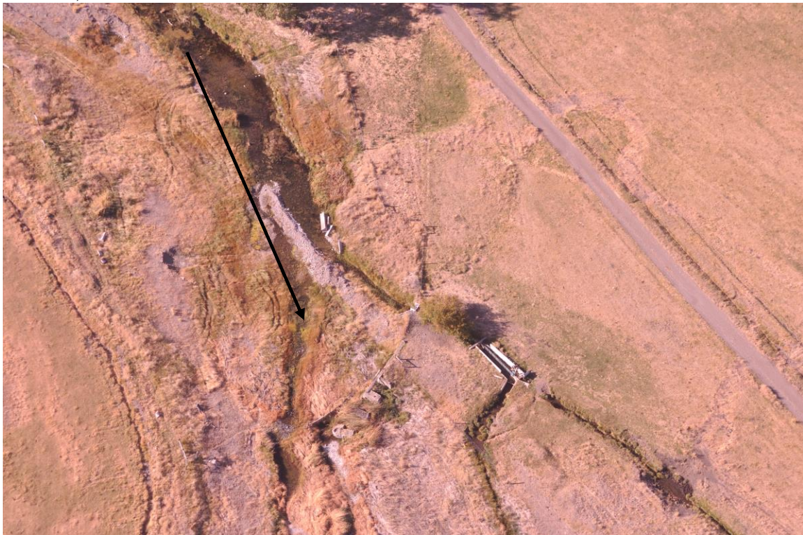
Photo 3, Parks Cr.diversion 4 on 10/18/12. The arrow shows the direction of flow
