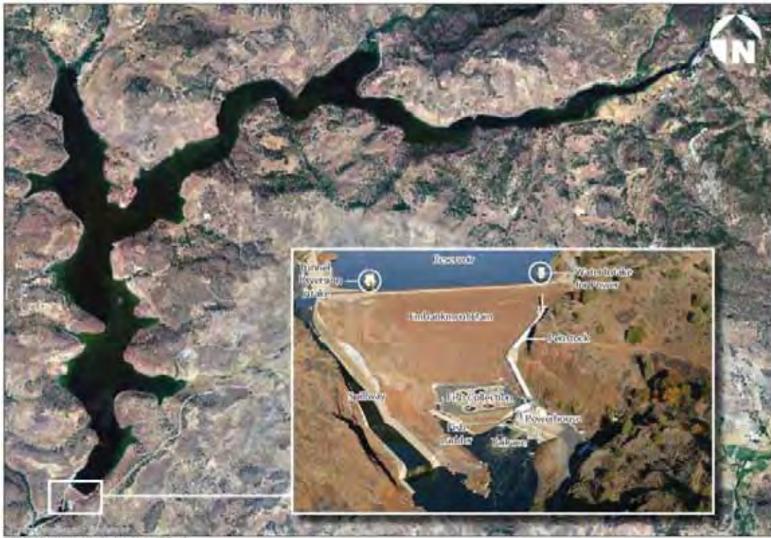
Figure ES-6. Iron Gate Dam, Reservoir, and Power Generating Facilities.
