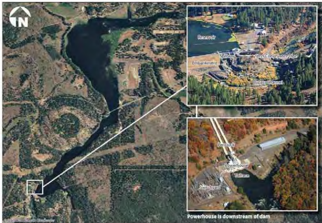
Figure 3.19-9. View of J.C. Boyle Powerhouse.
