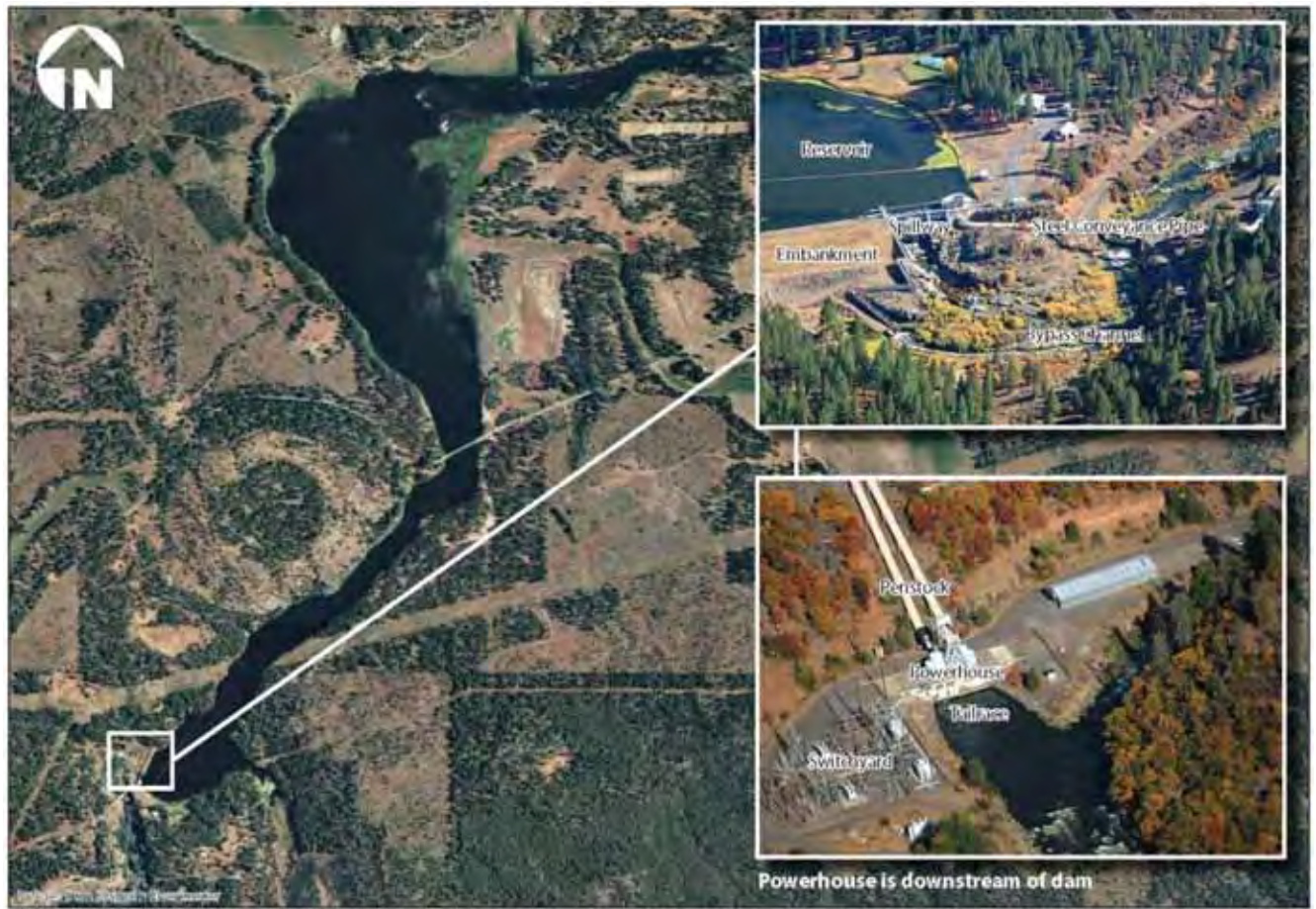
Figure 2-2. J.C. Boyle Dam and Powerhouse.
