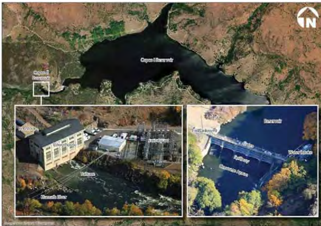
Figure ES-5. Copco 2 Powerhouse (left photo) and Dam.
