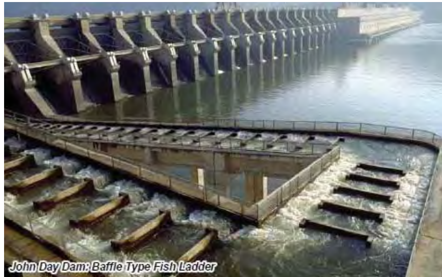
Figure 3.19-10. Example of cast in place pool and weir fish ladder used for fish passage, similar to that proposed for upstream fish passage for all four dams under this alternative.
