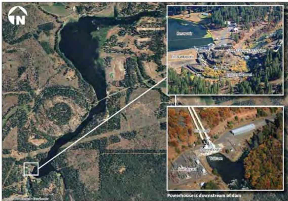
Figure ES-3. J.C. Boyle Dam and Powerhouse.
