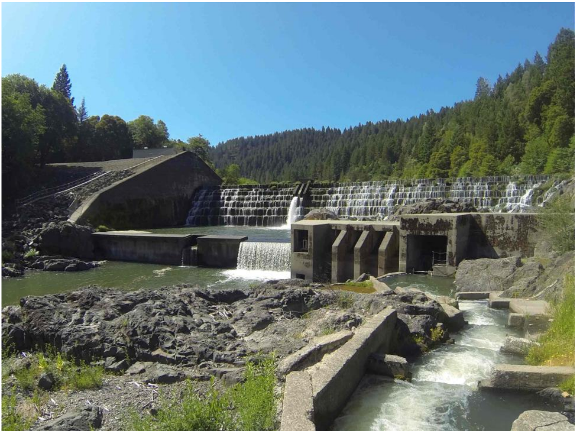
Figure 5. Van Arsdale Dam on the Eel River. The dam and fish ladder restricts passage of Pacific Lamprey to upstream reaches and is being used to study lamprey passage capabilities and test lamprey specific passage facilities.
