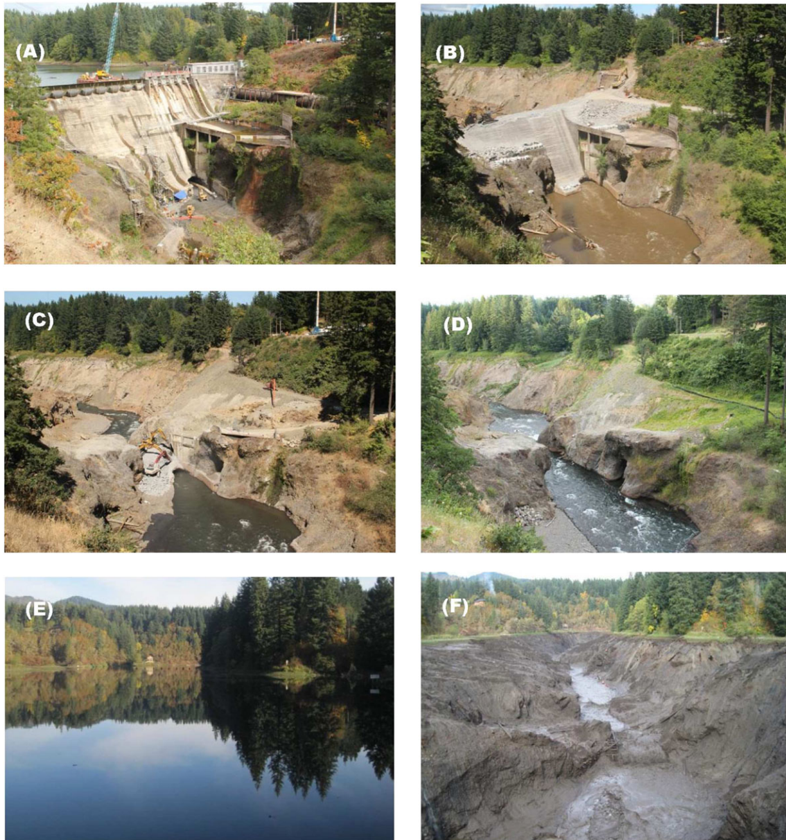
Figure 2. Decommissioning photos of Condit Dam as shown by photos taken by time-lapse cameras by Steve Stampfli of White Salmon, Washington. (A) The initiation of dam removal before the reservoir was drained, (B) approximately 75% decommissioned, (C) approximately 90% decommissioned, (D) 100% decommissioned. Photos (E) and (F) were taken by PacifiCorp staff on the day the reservoir was drained on 26 October 2011.
