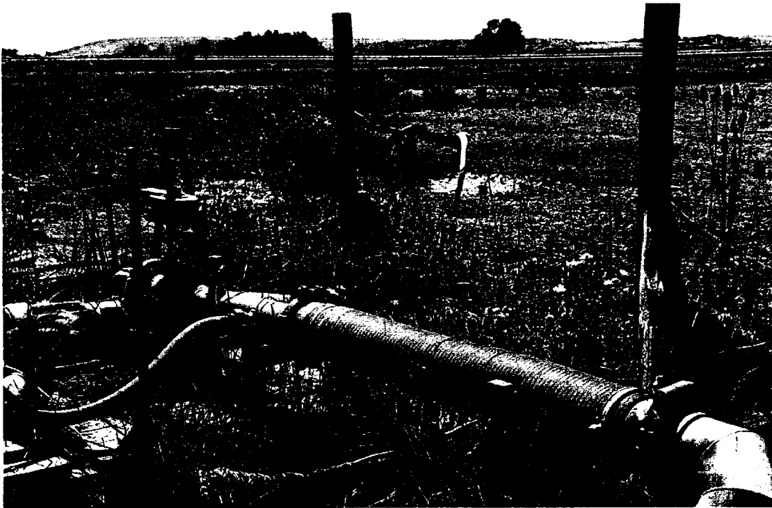
Figure A5-37. Pump installed at Fiock Ranch to eliminate the need for a diversion dam on the lower Shasta River. Dam removal should help improve dissolved oxygen conditions locally.
