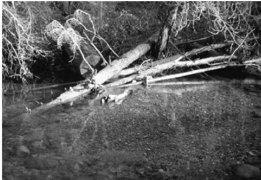
Figure A5-55. Complex log-cover structure in side channel of Elk Creek installed by Klamath National Forest. Photo courtesy of Al Olson. Circa 1991. Note spawning gravels adjacent to structure.
