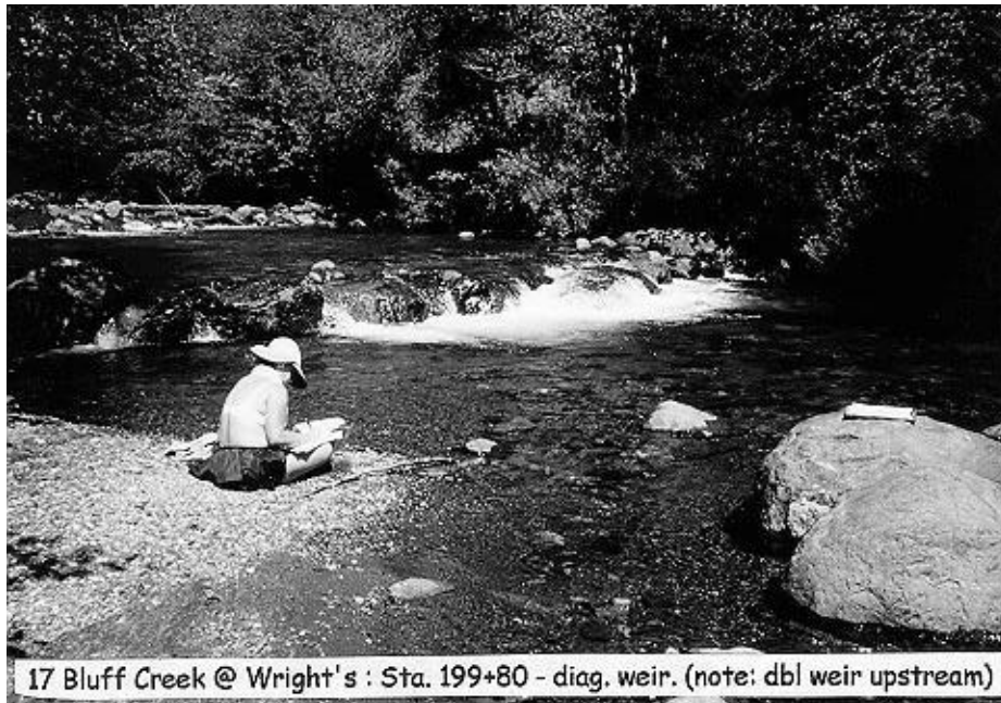
Figure A5-7. Boulder weir on Bluff Creek in September 1997. Photo courtesy of Six Rivers National Forest.
