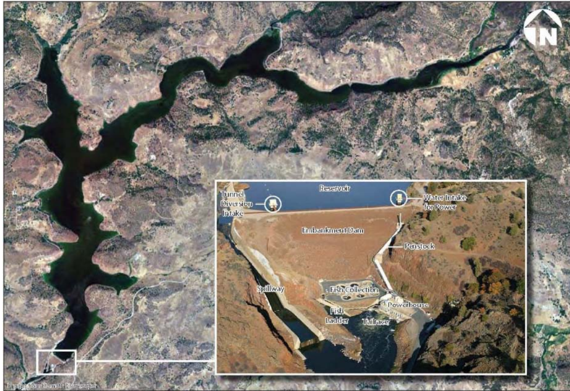
Figure 2-6. Iron Gate Reservoir, Dam, Fish Collection Facilities, and Powerhouse (Images from Klamath Riverkeeper)
