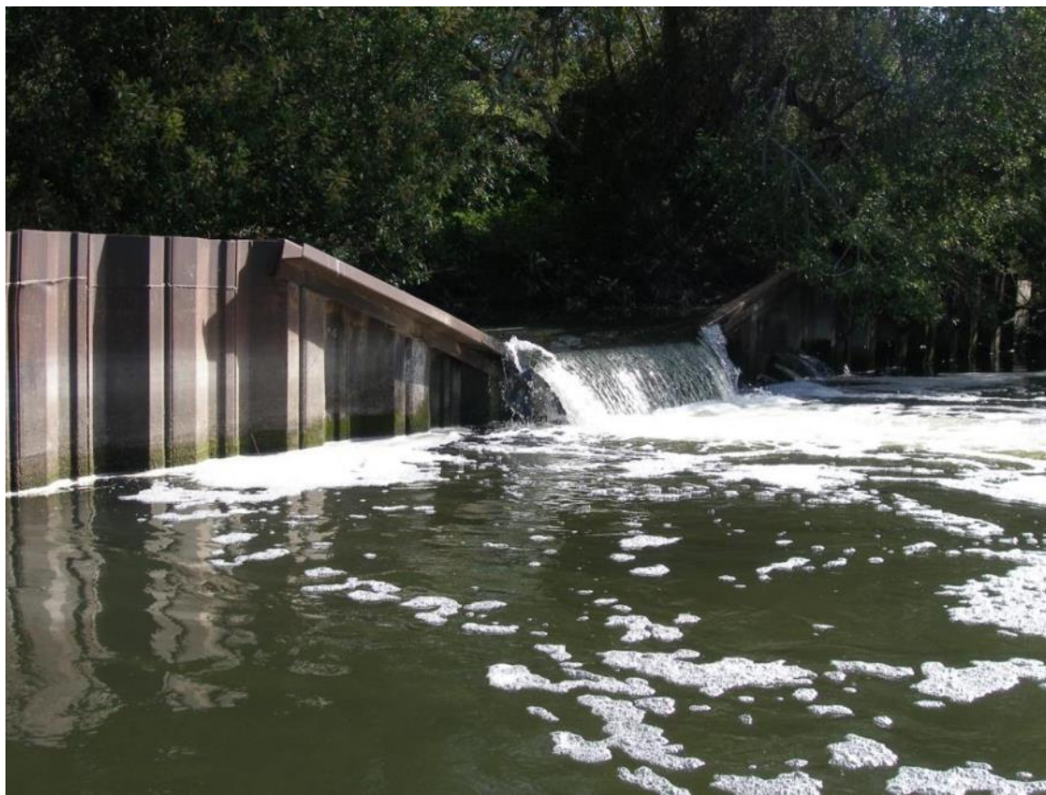
Figure 11. The Marre Tidal Weir at the San Luis Obispo Creek estuary. The weir was modified in 2006 to provide improved passage for coastal Rainbow Trout. Unfortunately, the design likely excluded Pacific Lamprey and may have extirpated the population. Photo taken in March 2012.
