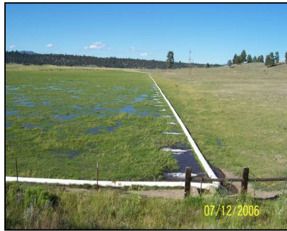
Figure 5. Photo of a Gated Pipe Irrigation System.
