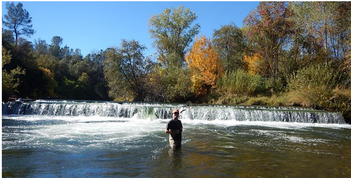
Figure 7. Sheetpile structure on lower Clear Creek to protect irrigation siphon below streambed. This structure may pose an obstacle to upstream lamprey migration and reduce their ability to reach upstream habitats.
