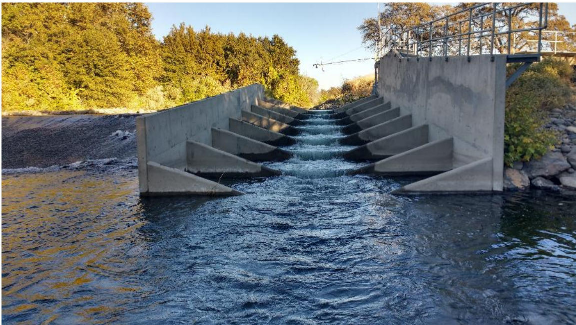
Figure 6. Ward Weir on lower Mill Creek with new lamprey-friendly fishway structure. Note weirs have rounded tops to provide lamprey climbing routes and are v-shaped to provide low velocity climbing routes at a range of streamflows. However, many other fish passage facilities in the Sacramento RMU do not provide lamprey friendly passage routes.
