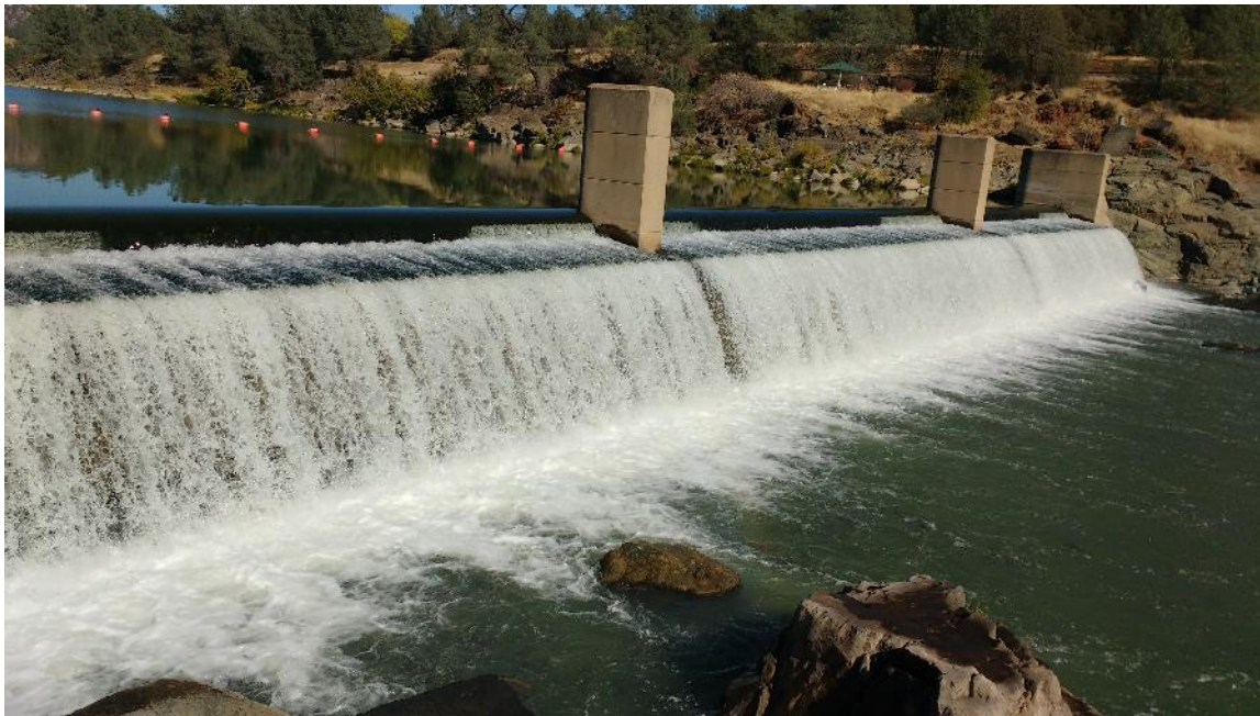
Figure 5. Fish Barrier Dam below Oroville Dam on the Feather River adjacent to the Feather River hatchery.
