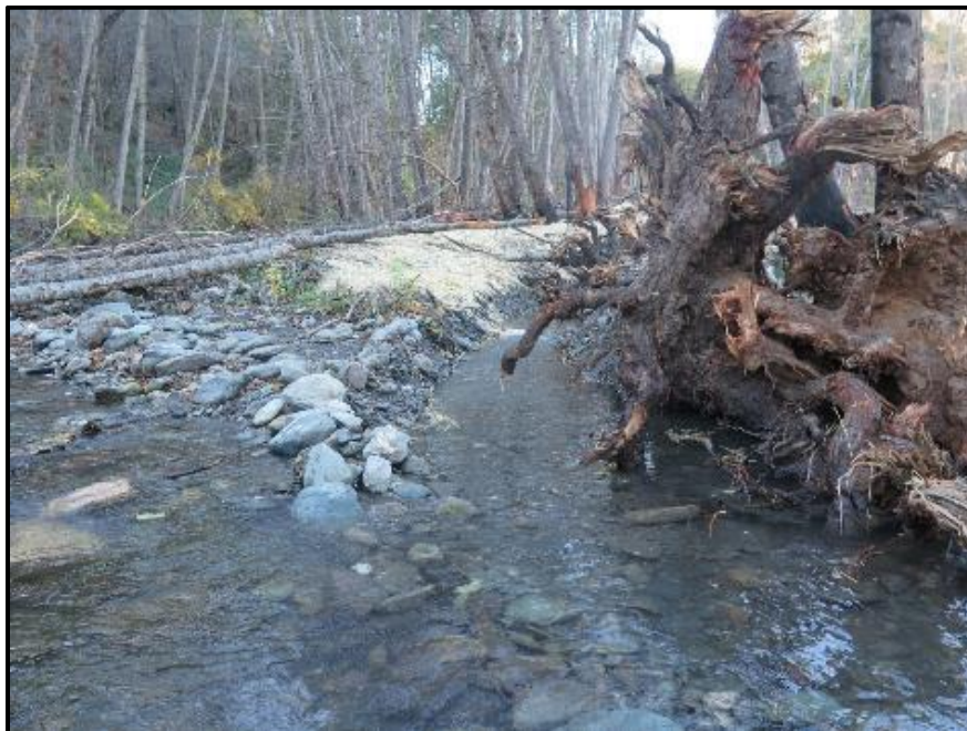
The Lawrence Ponds, constructed in 2017, shows the latest design iteration of an ingress-egress channel. The downstream junction angle of the channel and large wood installed at the confluence will help reduce seasonal deposition within the constructed channel.
