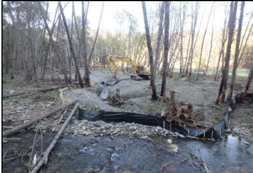
The Lawrence Ponds, constructed in 2017, shows the latest design iteration of an ingress-egress channel. The downstream junction angle of the channel and large wood installed at the confluence will help reduce seasonal deposition within the constructed channel.
