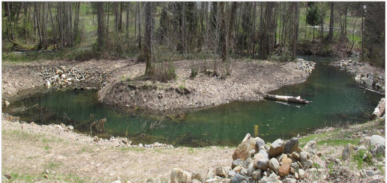
Figure 4. After construction of Alexander Pond, photographed in February 2011.
