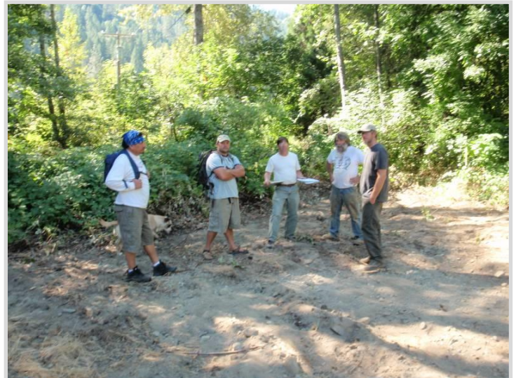
Figure 1. MKWC, Karuk Tribe, Fiori GeoSciences Inc., and the contractor review excavation plans (Sept, 2010) design concepts for Alexander Pond.
