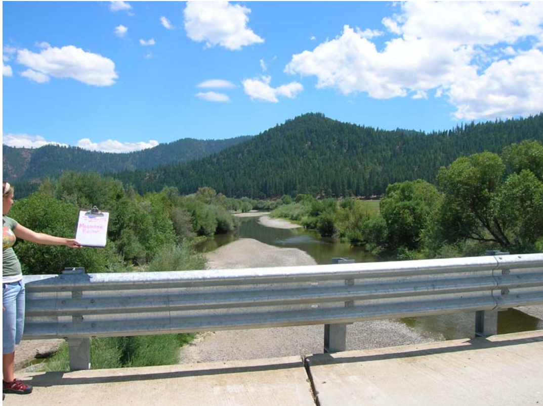
Figure 23- Scott River at Meamber Bridge looking upstream
