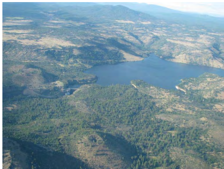
Figure 4.1-25: The relatively deep Copco 1 Reservoir experiences thermal stratification and results in low dissolved oxygen (from less than 1 mg/L to 5 mg/L) in reservoir bottom waters during summer and fall months. This poor water quality affects the Klamath River downstream of Copco 1 Dam.
