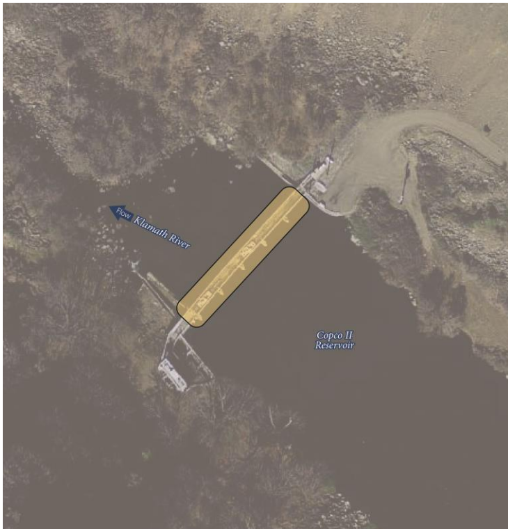
Figure 4.2-15: Partial removal of Copco 2 facility would provide a free flowing river and allow full volitional fish passage. However, certain structures would be retained.
