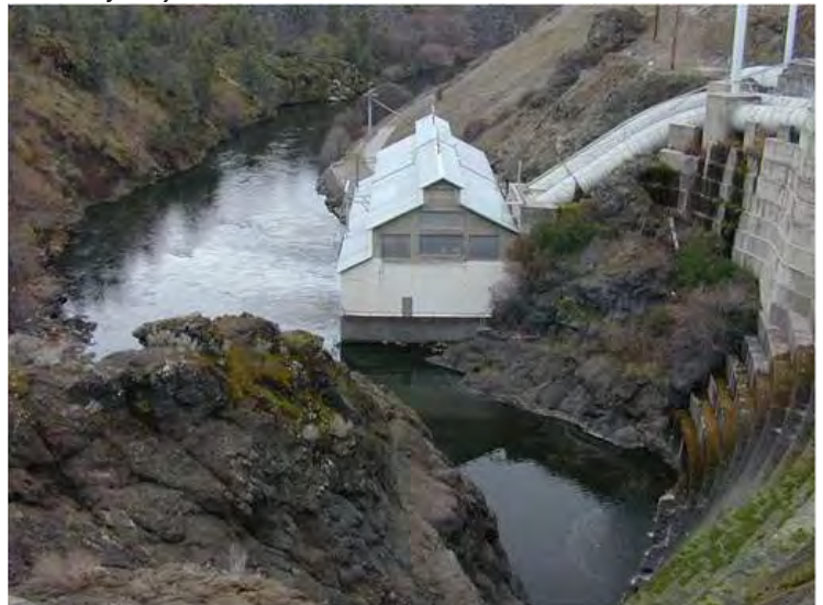
Figure 1-9: Copco 1 Dam, powerhouse, and downstream area of the Klamath River. This facility would be removed under the KHSA.
