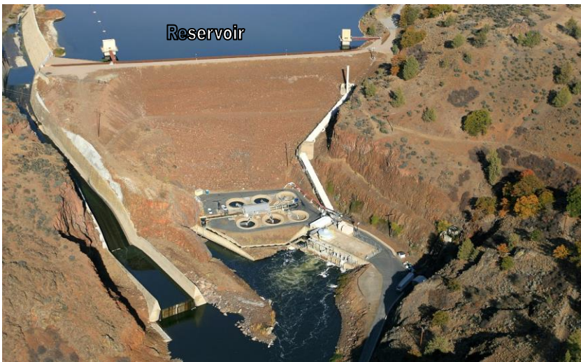
Figure 4.2-16: Photo of Iron Gate Dam and reservoir with specific components labeled. With full facilities removal, all visible components would be removed. With partial facilities removal, certain components (e.g., penstock) would be retained.
