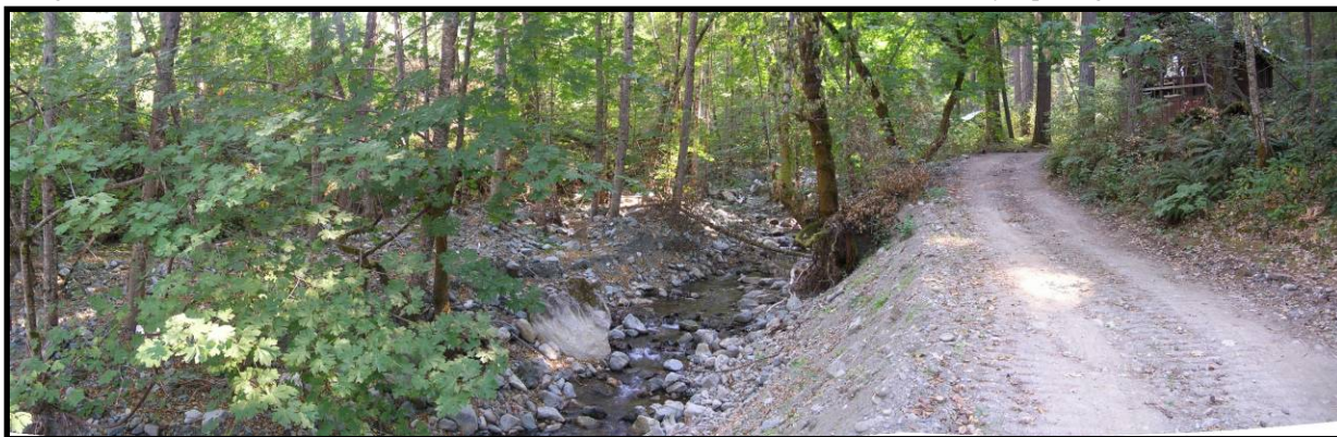
Figure 28. Private roads encroach on critical sections of Mid-Klamath tributaries, chronically inputting sediment.
