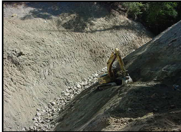
Figure 32. Road decommissioning in Steinacher Creek.
