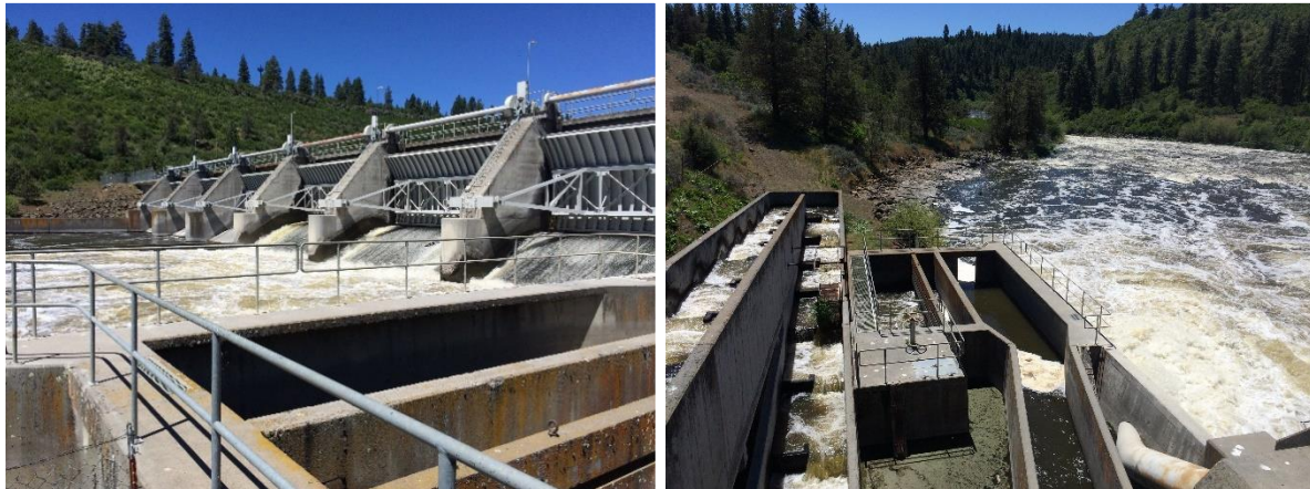
Figure 3-12. Keno Dam (left) located at rkm 380.5 (rm 236.4) with radial arm gates that draw water from below the surface. Keno Dam fish ladder (right) with attraction flow occurring to the side of the ladder entrance.
