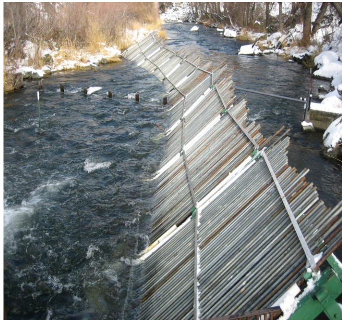
Figure 3: Alaska-style panels of the Shasta River Fish Counting Facility (SRFCF)
