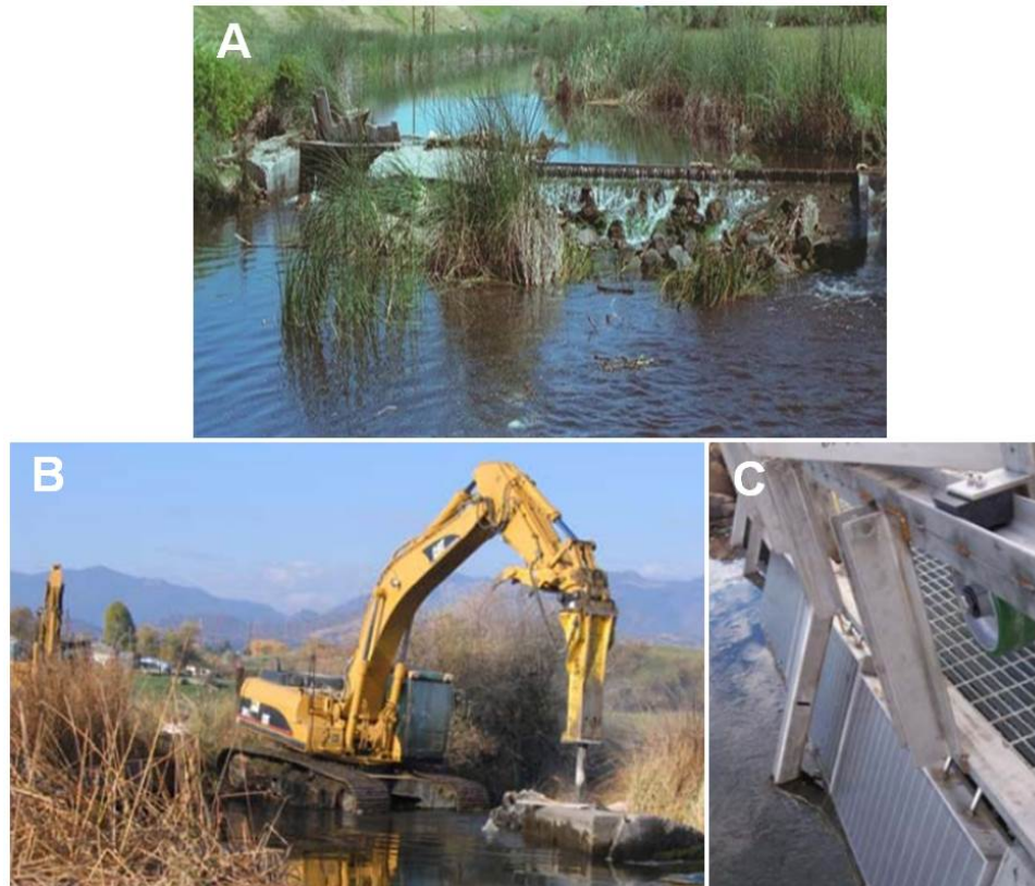
Figure 6-14: The Araujo Dam prior to (A), during (B), and after removal (C) when it was replaced by a screened diversion pump (Unkefer 2008).
