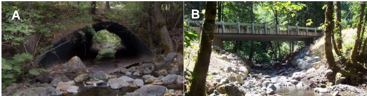
Figure 6-13: Road crossing at Whites Gulch before (A) and after (B) fish passage project (Five Counties 2010). Sources of data and methods described in Appendix H.
