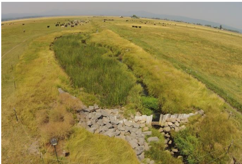
Figure 6-43: A photo of one of the diffuse source treatment wetlands (DSTW) that was constructed on Sevenmile Creek, along with riparian fencing to keep out livestock. Reproduced with permission from Trout Unlimited.
