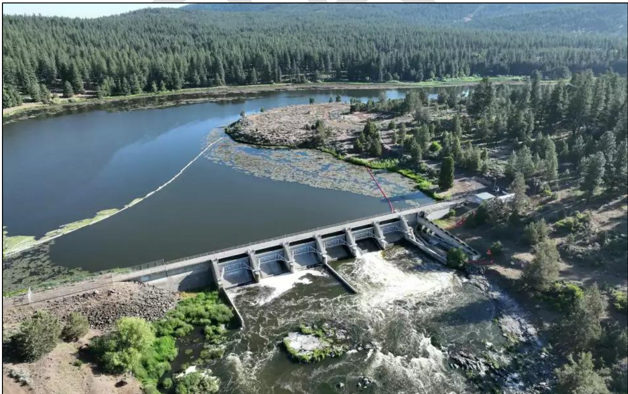
Figure 5. Link River Dam (upper photo) and Keno Dam (lower photo).
